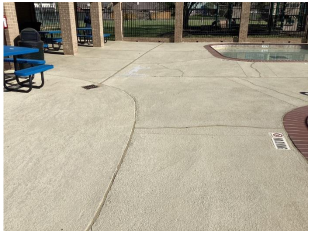
Concrete pool deck overview
