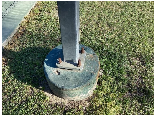
Rusted fasteners
