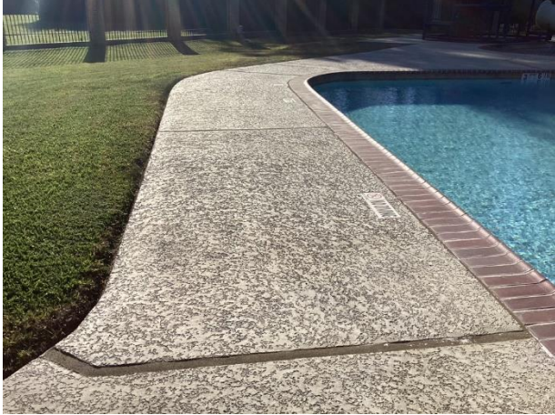
Concrete pool deck overview
