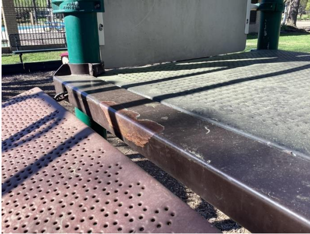
Equipment finish deterioration
