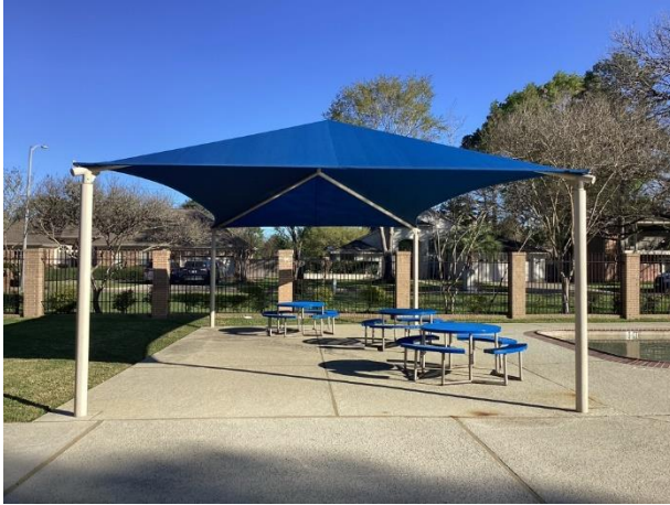
Shade structure overview
