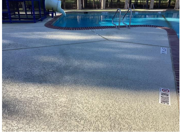
Concrete pool deck overview
