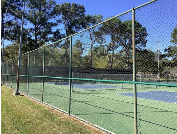
Chain link fence
