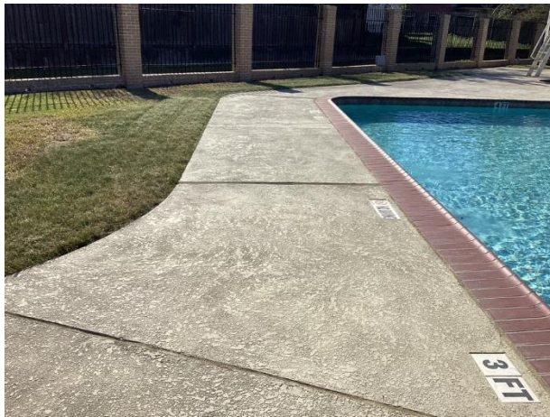
Concrete pool deck overview
