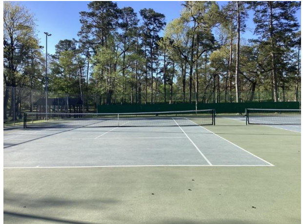
Tennis court overview
