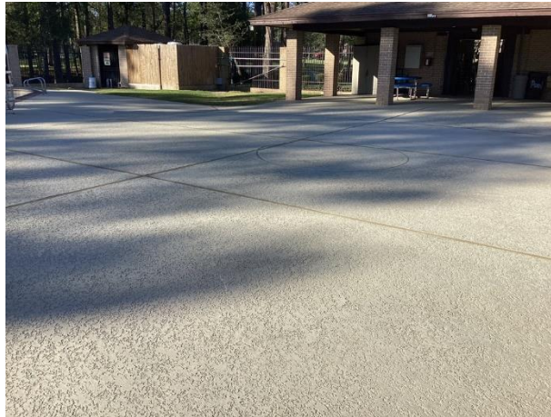
Concrete pool deck overview
