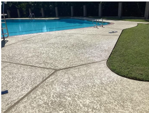
Concrete pool deck overview
