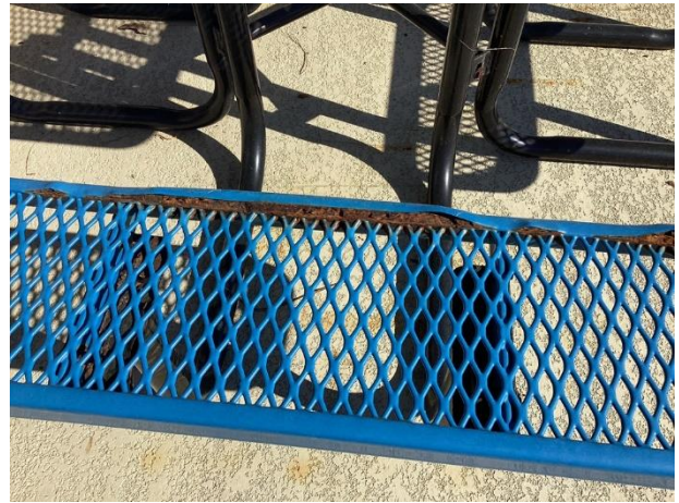
Site furniture with rust and deterioration
