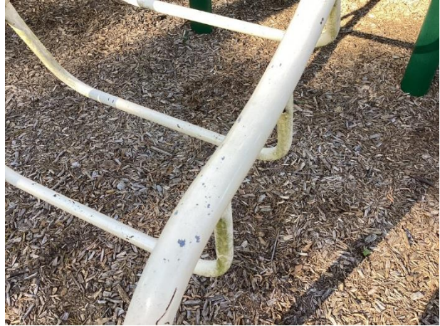
Equipment finish deterioration
