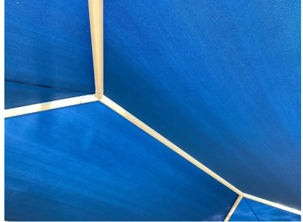
Shade structure overview
