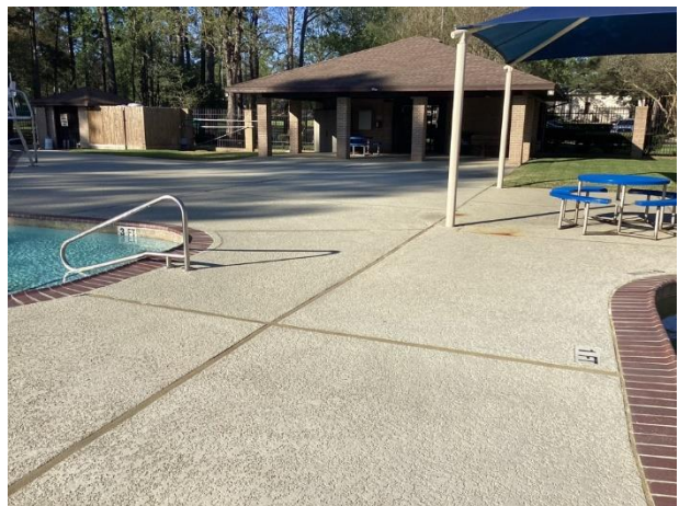
Concrete pool deck overview
