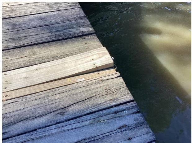
Warped board
