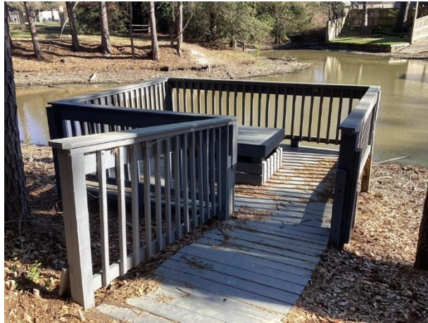
Dock with wood decking
