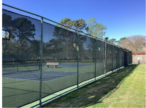
Chain link fence
