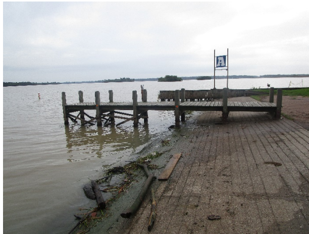
Wood dock overview
