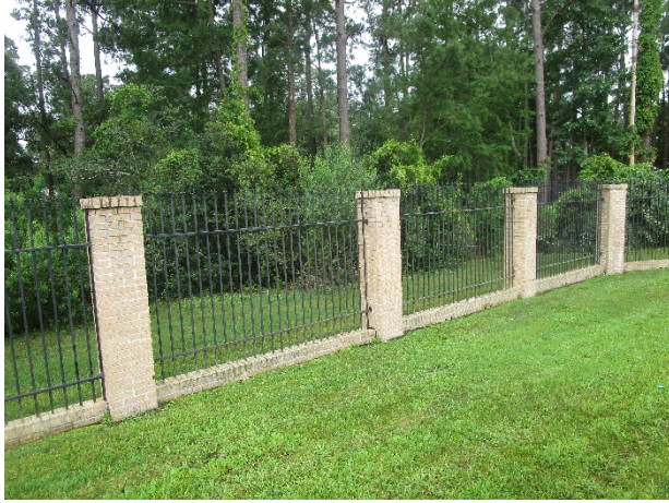
Metal pool fence overview
