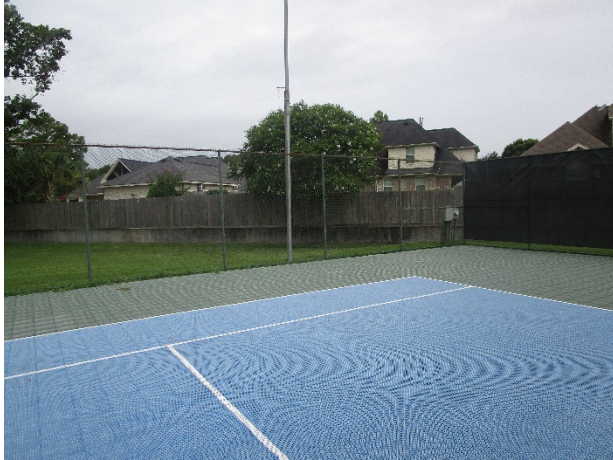
Pinehurst tennis courts fence overview
