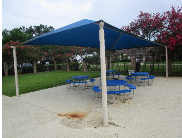
Shores pool shade structure
