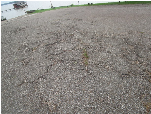
Pavement cracks
