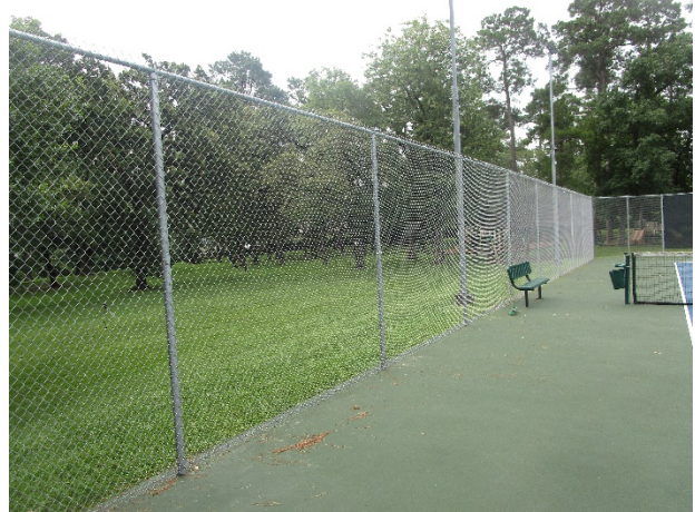
Shores tennis courts fence overview
