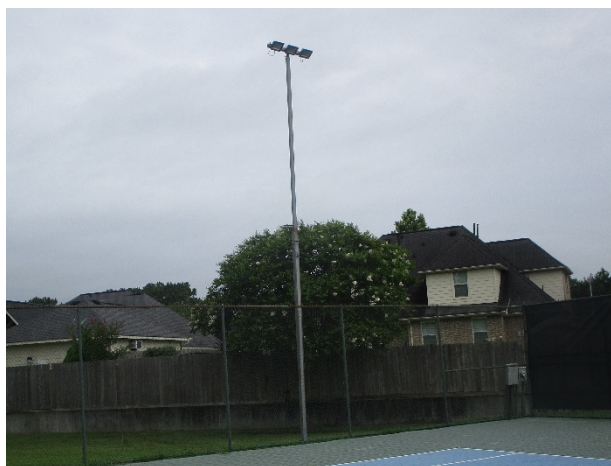
Tennis courts light pole and fixture overview
