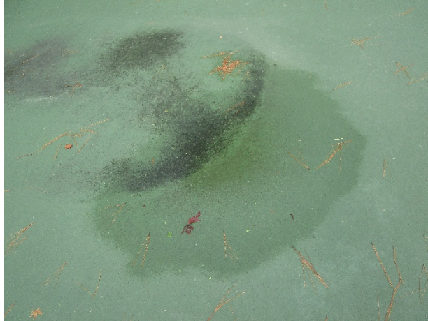
Color coat deterioration
