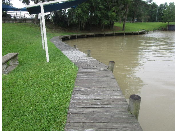
Wood walkway overview
