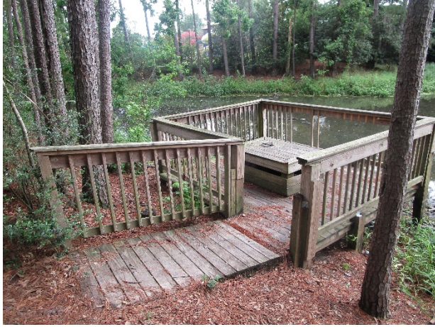
Wood dock overview
