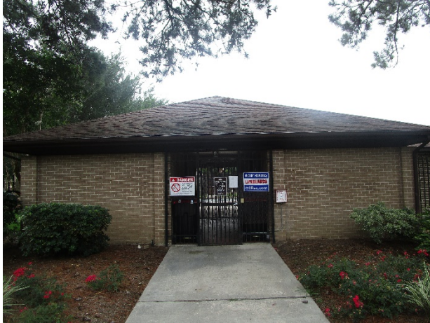
Asphalt shingle roof overview
