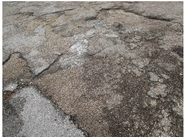
Pavement deterioration
