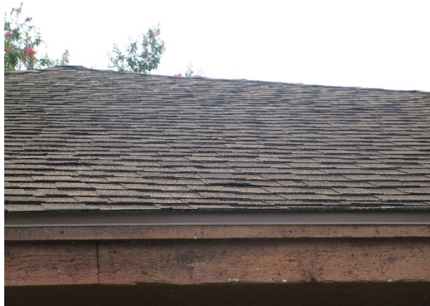
Shingle lift at the Shores pool house roof
