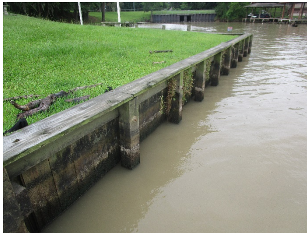
Timber bulkhead overview
