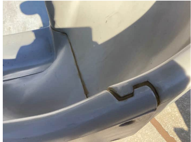
Recently replaced sealant in good condition
