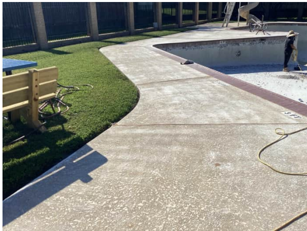
Concrete pool deck overview at Pinehurst
