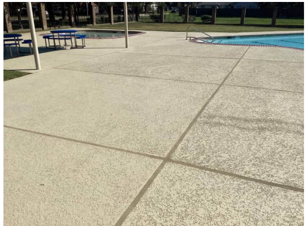
Concrete pool deck overview at Shores
