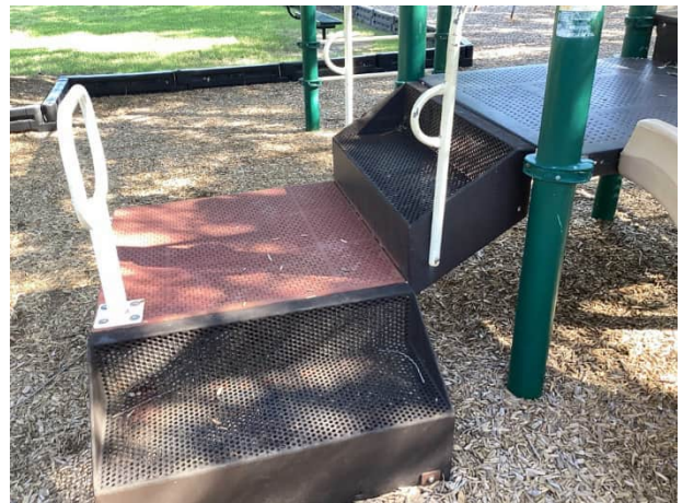
Recently replaced platform
