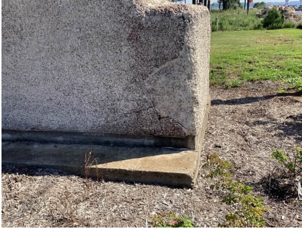
Concrete cracks
