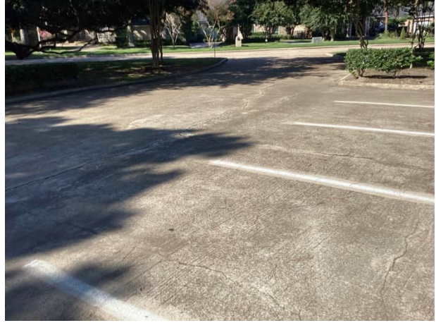
Parking area overview
