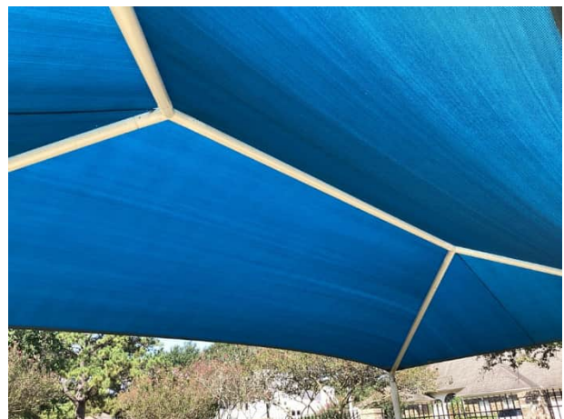
Shade structure overview
