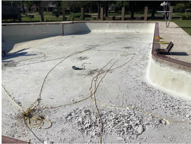
Pinehurst pool plaster overview
