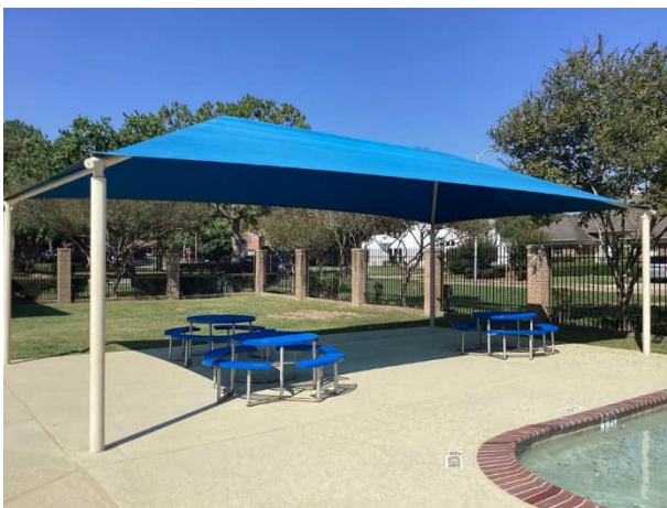
Shade structure overview
