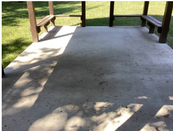
Gazebo concrete floor
